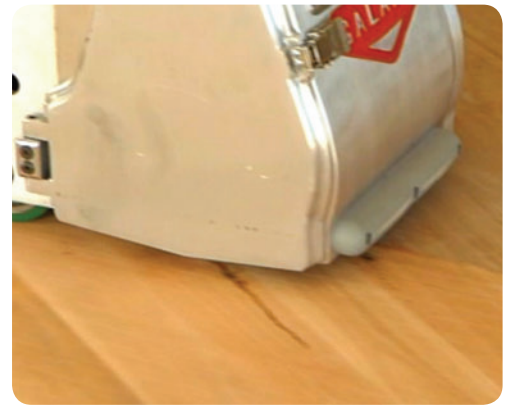
First pass of sanding at 45° to board direction.
