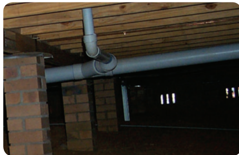
Adequate sub-floor ventilation and a dry sub-floor space are a must for timber floor performance.
