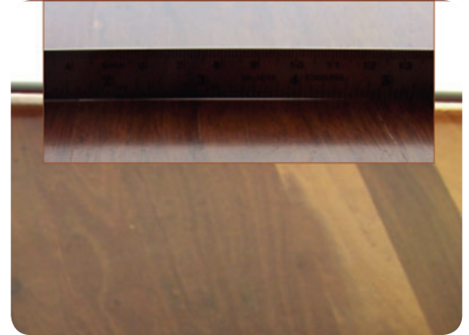
Cupping – Board edges higher than the centre of the board, but which is barely visible in the floor.
