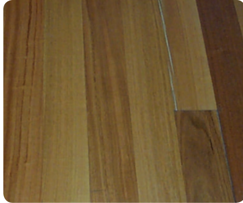
Edge bonding can result in wide irregularly-spaced gaps at board edges and split boards within the floor.
