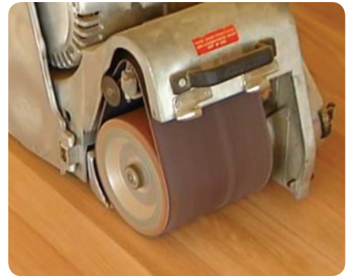
Third pass of sanding in the board direction.
