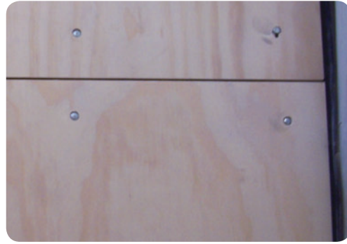
Plywood mechanically fixed to concrete.
