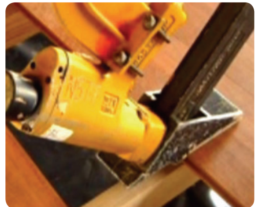
Secret fixing is recommended for boards up to 85 mm in cover width.
