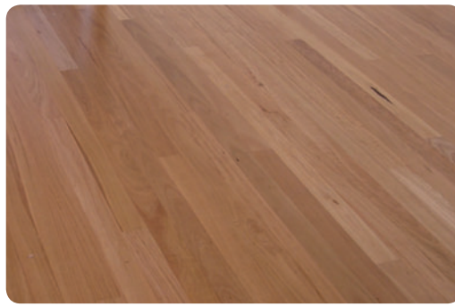
A select grade Blackbutt floor where the backsawn gum vein toward the top right exceeds grade limits but is acceptable within the floor.
