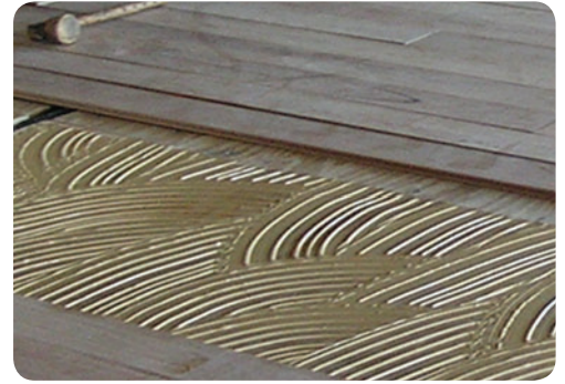
Adhesive spread prior to fixing.
