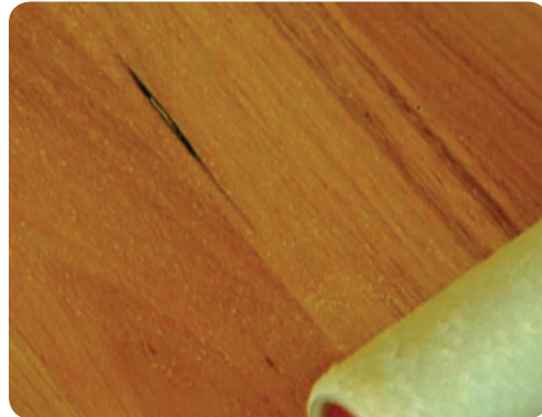
Application of the second coat.
