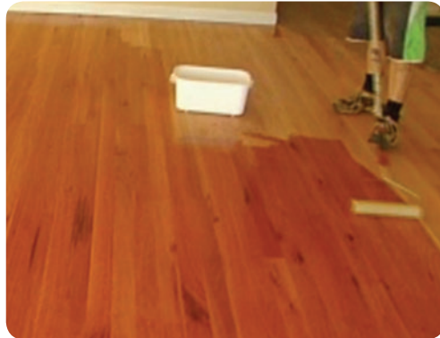
Application of the initial coat.
