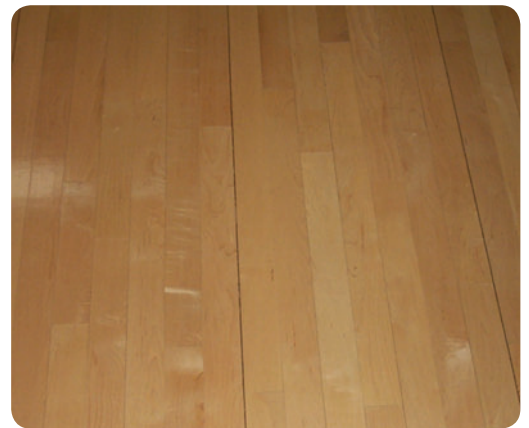
Particularly for wide floors or in moist climates small regular gaps can be used to provide the additional expansion allowance needed. These often close during humid periods.
