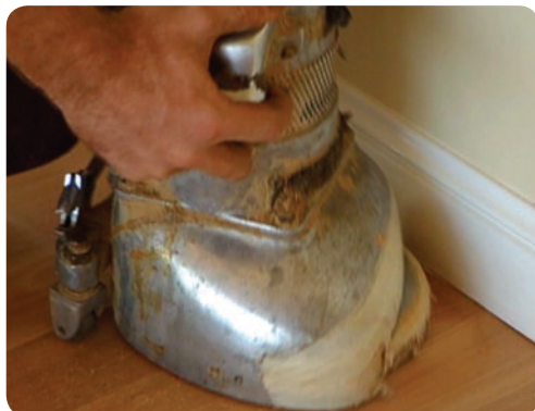
Edge sanding requires a smooth action to blend into the floor.
