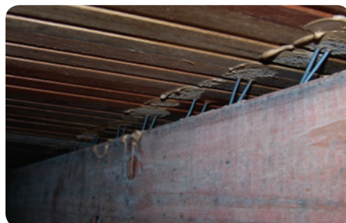
Buckling of 80 mm wide Spotted Gum boards secretly fixed to pine joists in a humid locality.
