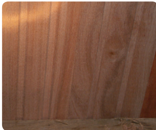
It should be checked that boards are tight on the joists.
